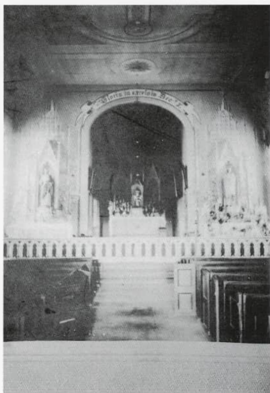
Interior of first brick church - built 1878.
