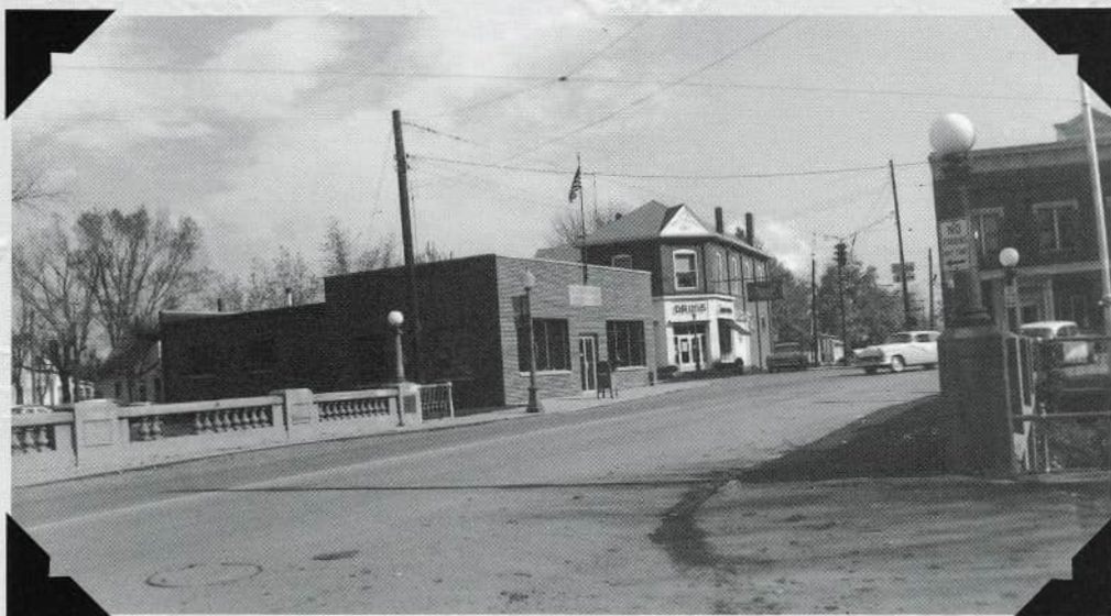
Post Office (center) Bridge crossing Miami-Erie Canal (Built by WPA)
