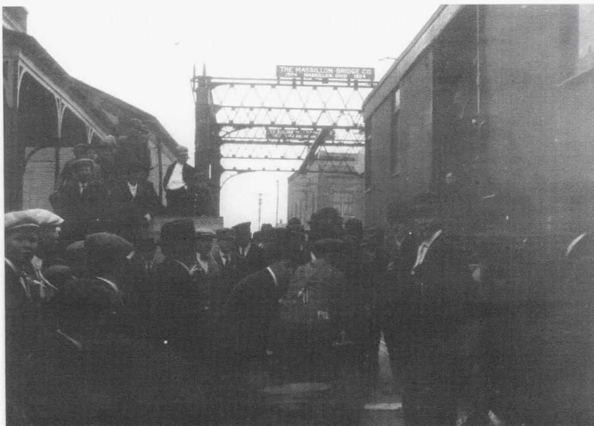
Monroe Street Bridge Photo Courtesy of Mark Renwick
