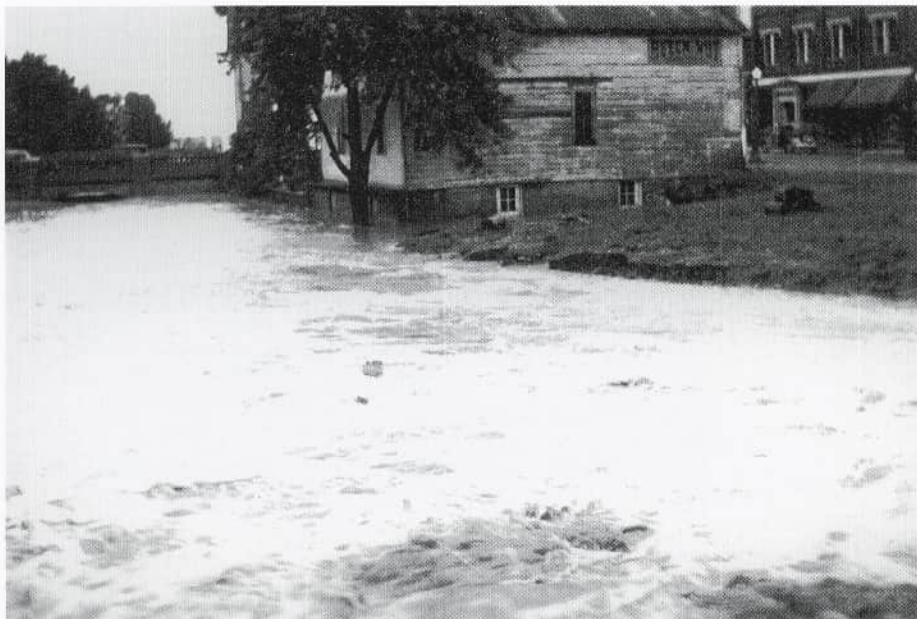
Monroe Street Bridge facing north Photo Courtesy of Ferd Wint
