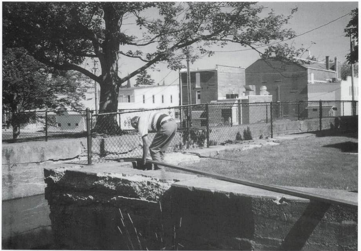
Deterioration of Lock One Photo Courtesy of Genevieve Conradi (2004)
