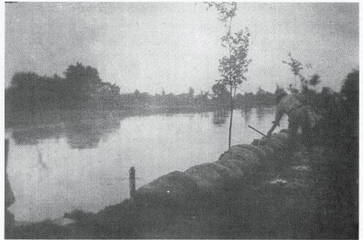
Placing sandbags on the canal bank near Comb's Ice House Photo Courtesy Paul A. Lietz Collection
