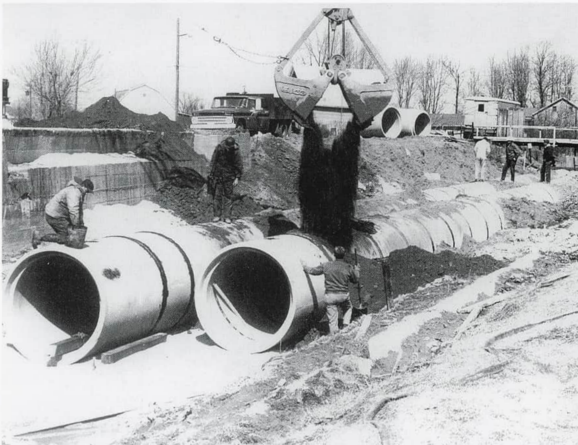
The canal was flumed under Monroe Street in 1968.
