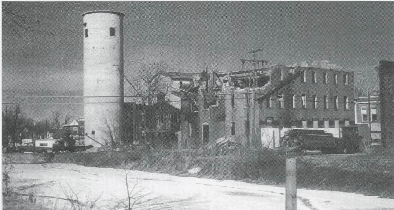
Mill being demolished Photo Courtesy of the Stan and Donna Mae Kuenning Collection
