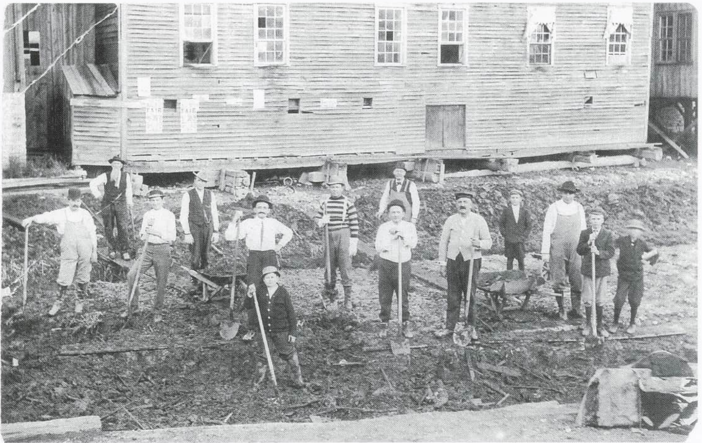
Workers with Shovels Photo Courtesy of Tom Fledderjohann
