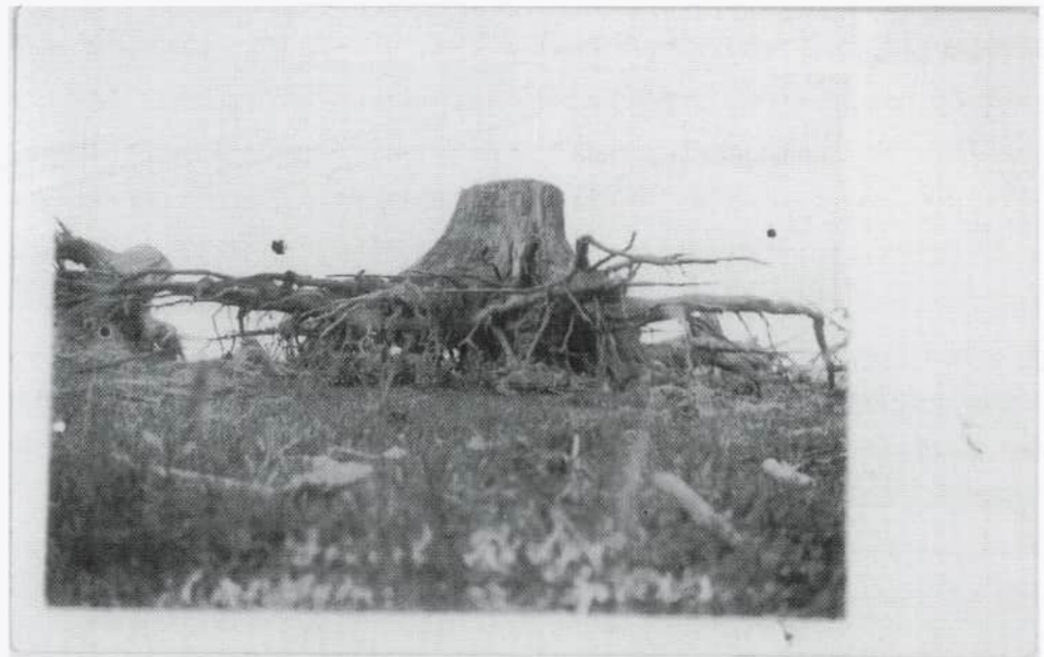
Technique for removing stumps Photo Courtesy of Tom Fledderjohann
