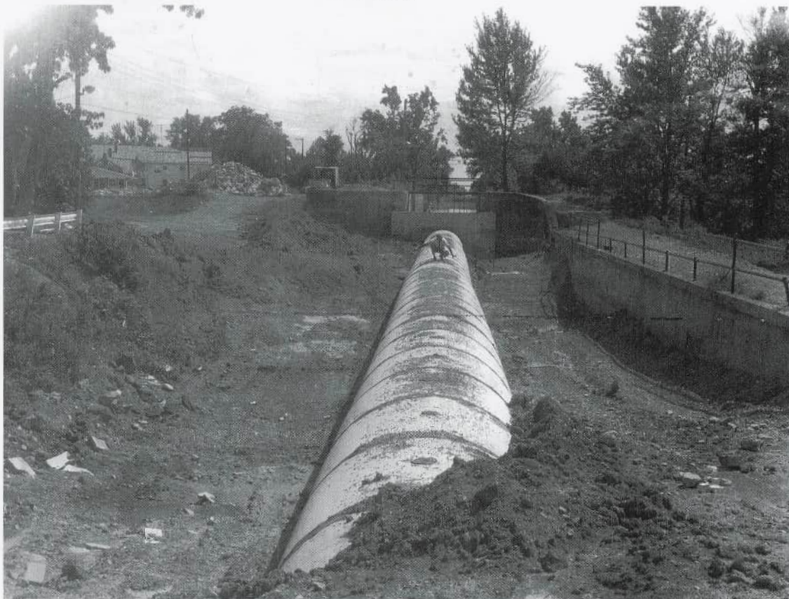
Fluming the Canal Lower Level of Lock One Photos Courtesy of the Village of New Bremen
