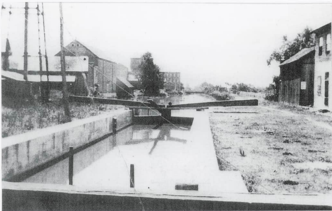
New Bremen Lock One North after concrete replacement in 1910. Photo by Ward Pape from the Collection of Jim Cooper
