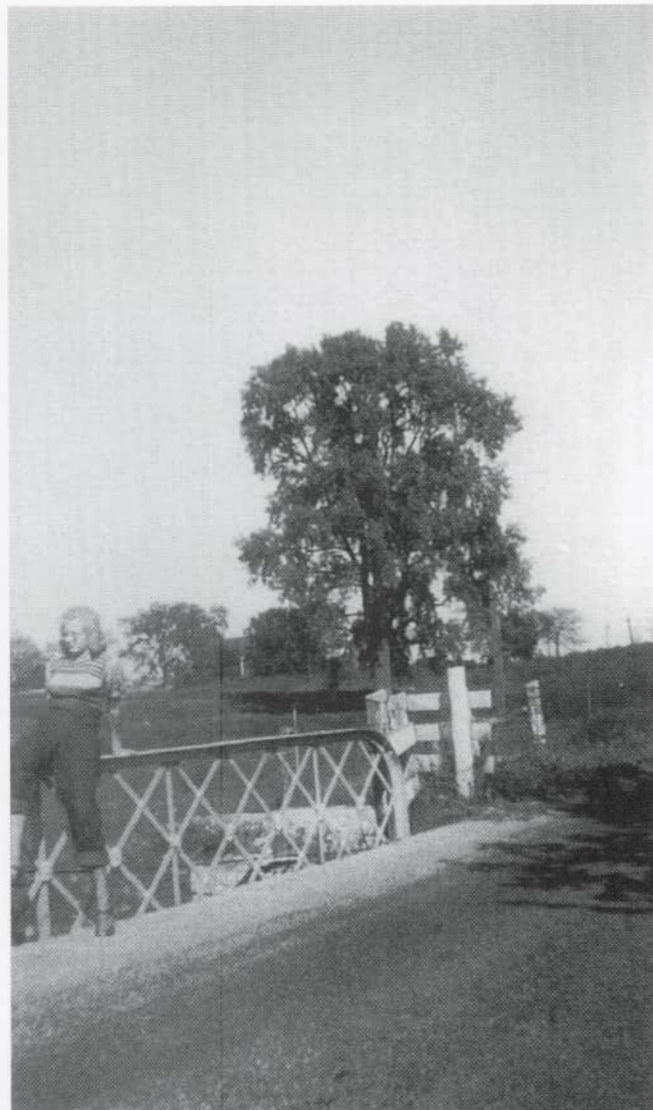
Lock Two Bridge Photo Courtesy of Delores Stienecker
