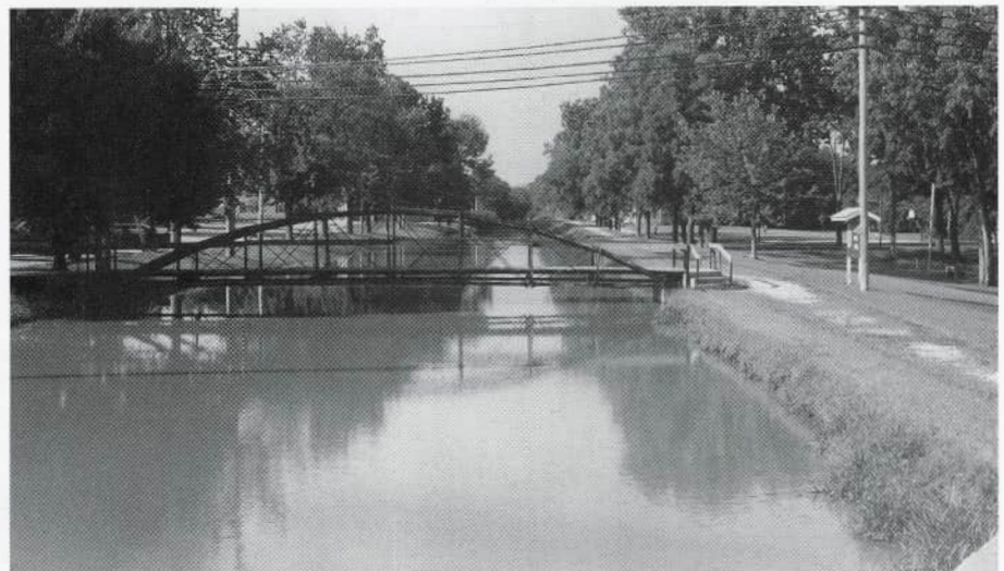
1864 Cast Iron Bridge Oldest Bowstring girder bridge in Ohio Photo Courtesy of Genevieve Conradi (2003)
